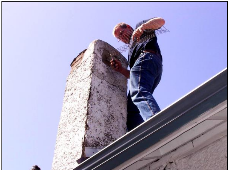
above pictures: Mr. Gerhard Oberauer installing protection wire for the bell tower and the chimney
