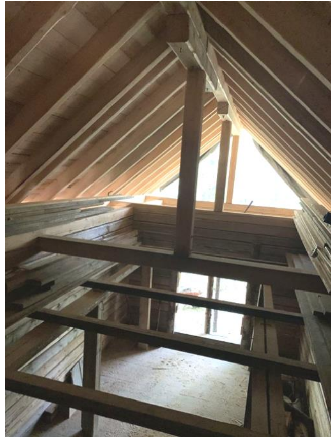
Interior construction of the Old Catholic Chapel (St. Hubert)
